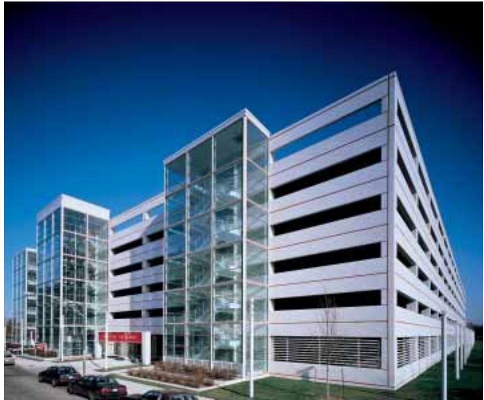
Cook County Juvenile Center Parking Garage, Chicago, IL Photo: William Kildow Photography
