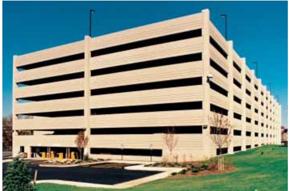
Station Plaza Parking Garage, Trenton, NJ
